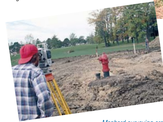
Manhard surveying crews collect and feed raw data to in-house surveying teams for processing. The output guides many activities at the job site, from erosion control to construction staking to earth moving.
